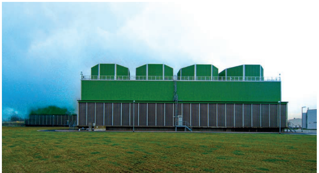
Cooling tower (courtesy Fiberline Composites)
