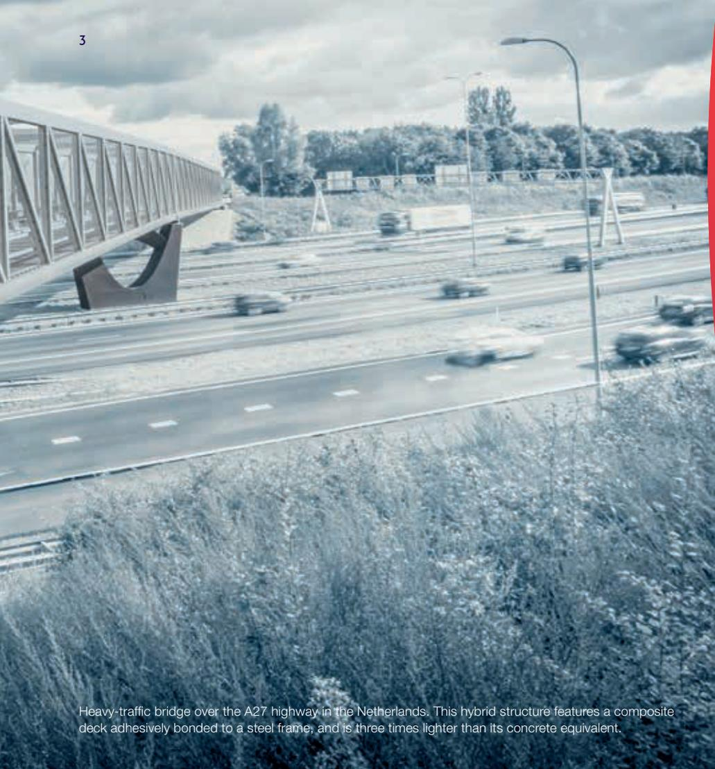
Heavy-traffic bridge over the A27 highway in the Netherlands. This hybrid structure features a composite deck adhesively bonded to a steel frame, and is three times lighter than its concrete equivalent.
