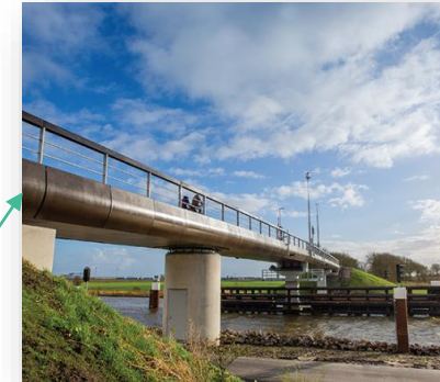
Bio-composite bridge 70m long Biobased 1800 ECO & flax Netherland
